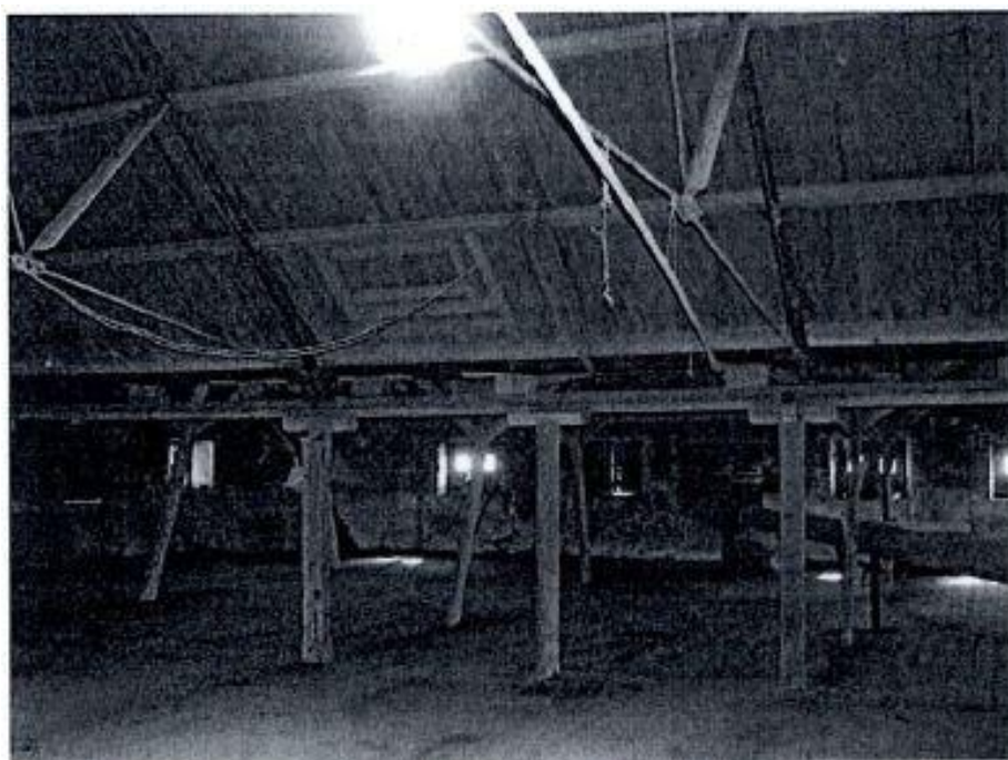
Malt House Interior - Roof Structure.
