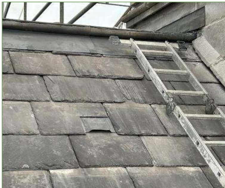
Plate 5.2 - Example of a lead bat access tile (Photo: Tom O'Donnell).
