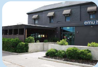
The Emu Hotel in Morphett Vale, South Australia, was one of 11 hotels added to our network in F23.
