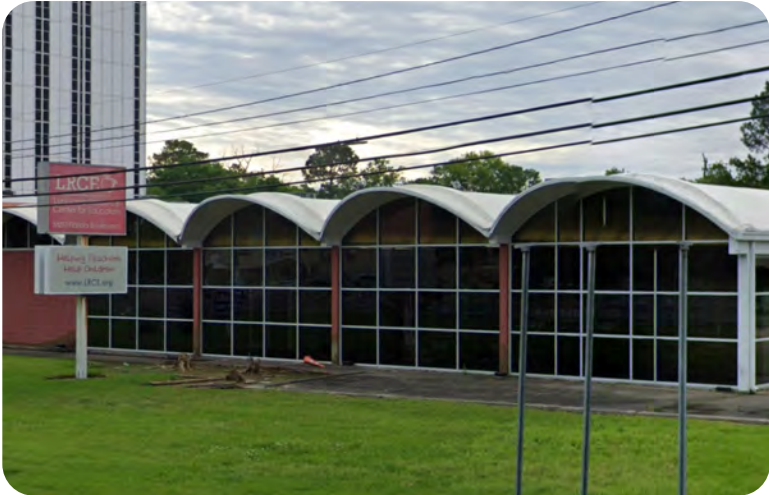
3.1 5550 Florida Blvd, LA Resource Center
