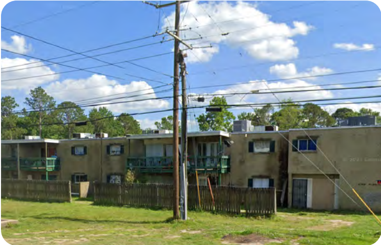
3.4 5750 Florida Blvd, River Pine Apartments
