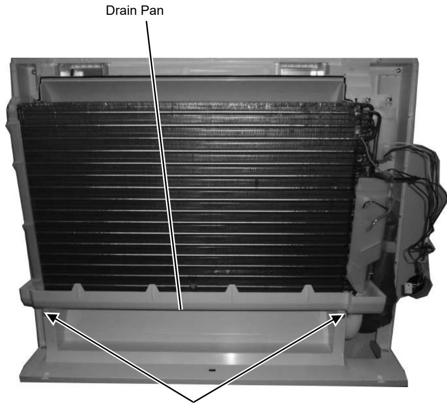
1. Release the 2 screws to remove the Drain Pan.
