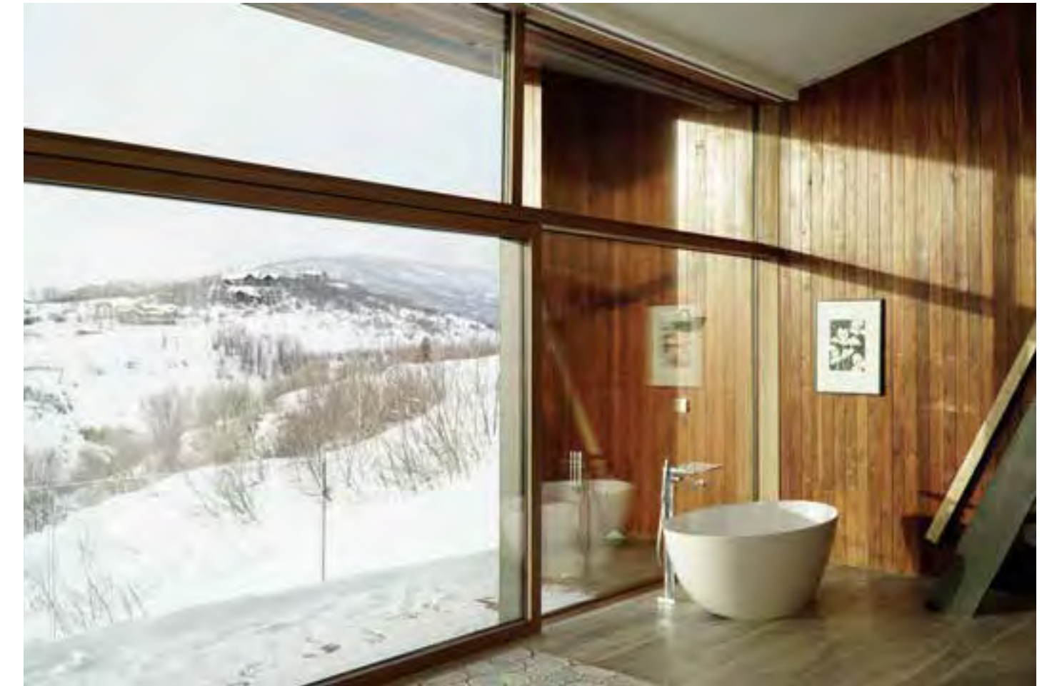
This Zola LiftSlide spans 48', including a post-less corner. The 10' height opens the view to Emerald Mountain.
