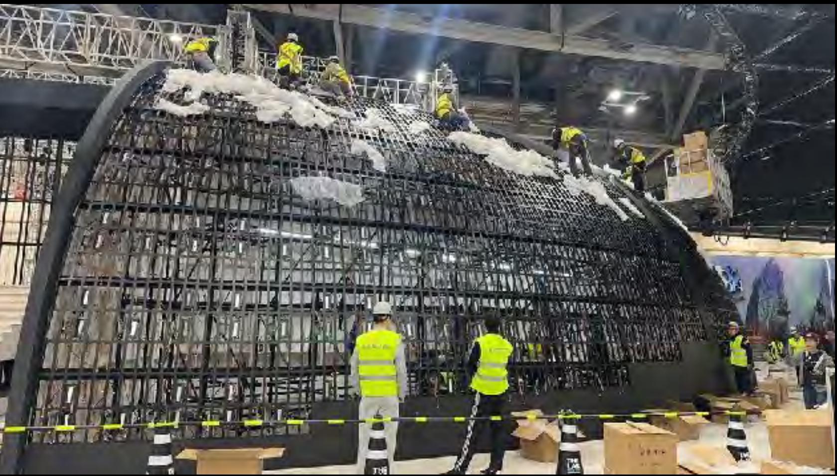
Prior to installation, a rehearsal is conducted to confirm that all structural components are correctly fabricated in line with the design.
