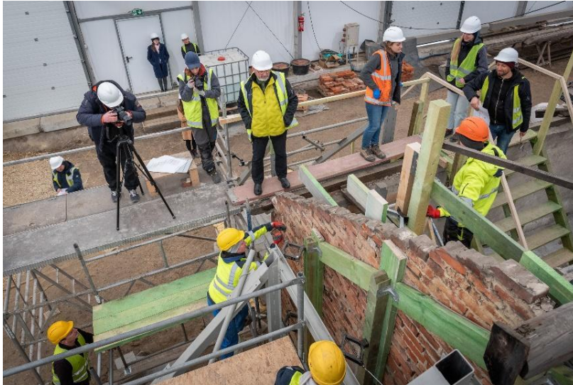
Photo 10. B-115 – straightening of the eastern wall (photo by R. Pacek)
