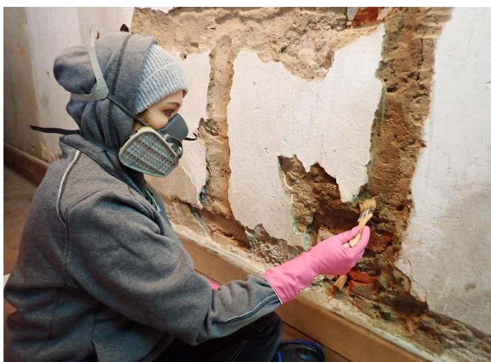
Photo 4. Plaster protection works (photo by J. Krasowska)
