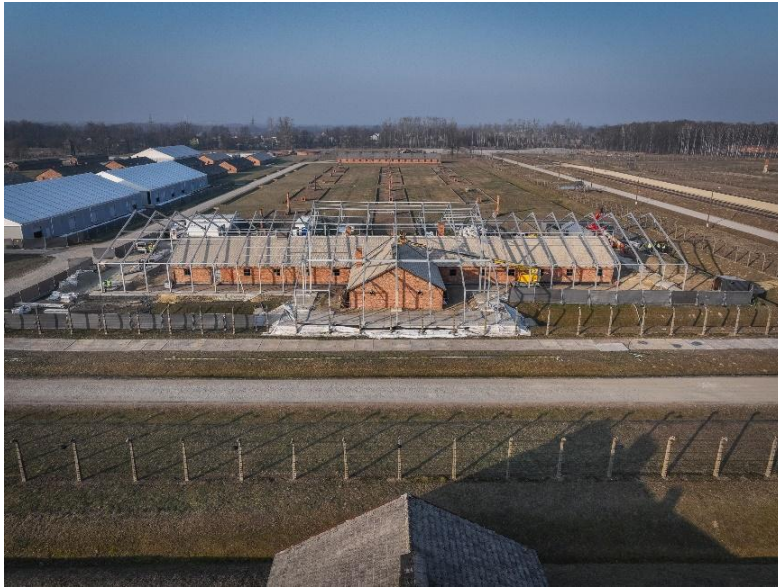
Photo 7. Dismantling of the protective structure above B-112 (photo by R. Pacek)
