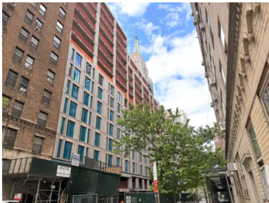
Facade installation progressing at The Morgan (May 2026)
