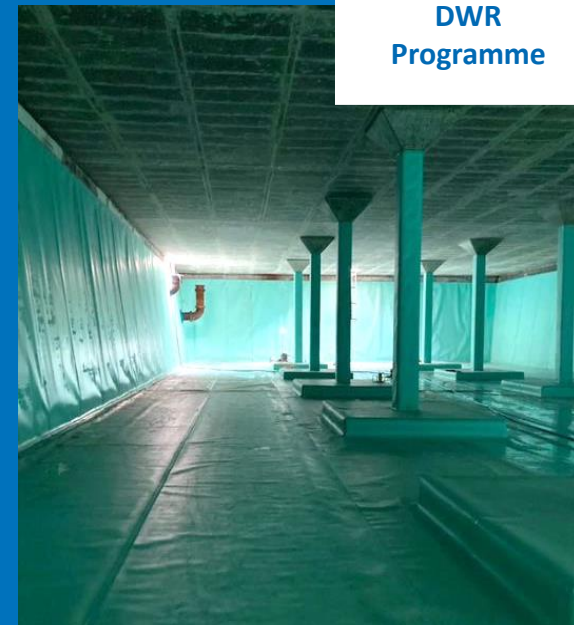
Hendrefydd SRV - Internal liner installation
