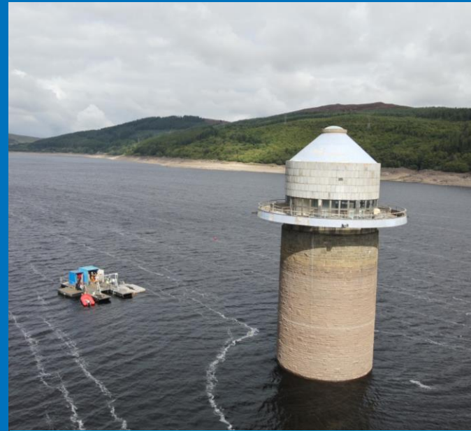
900mm Pipework installed
