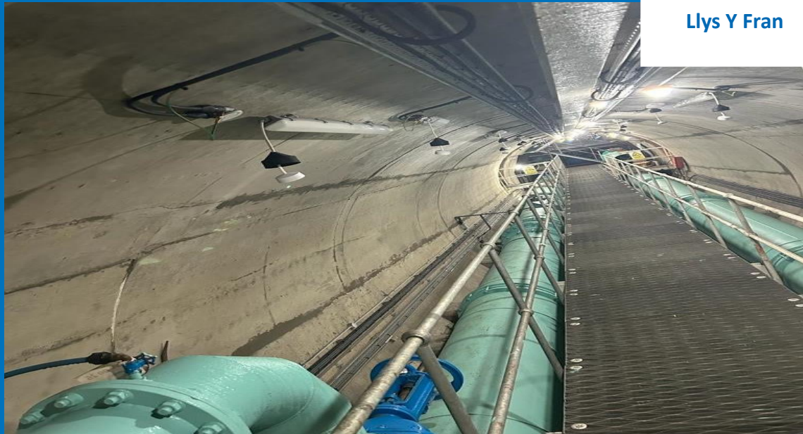
Newly Painted Valve and Pipework and new lighting
