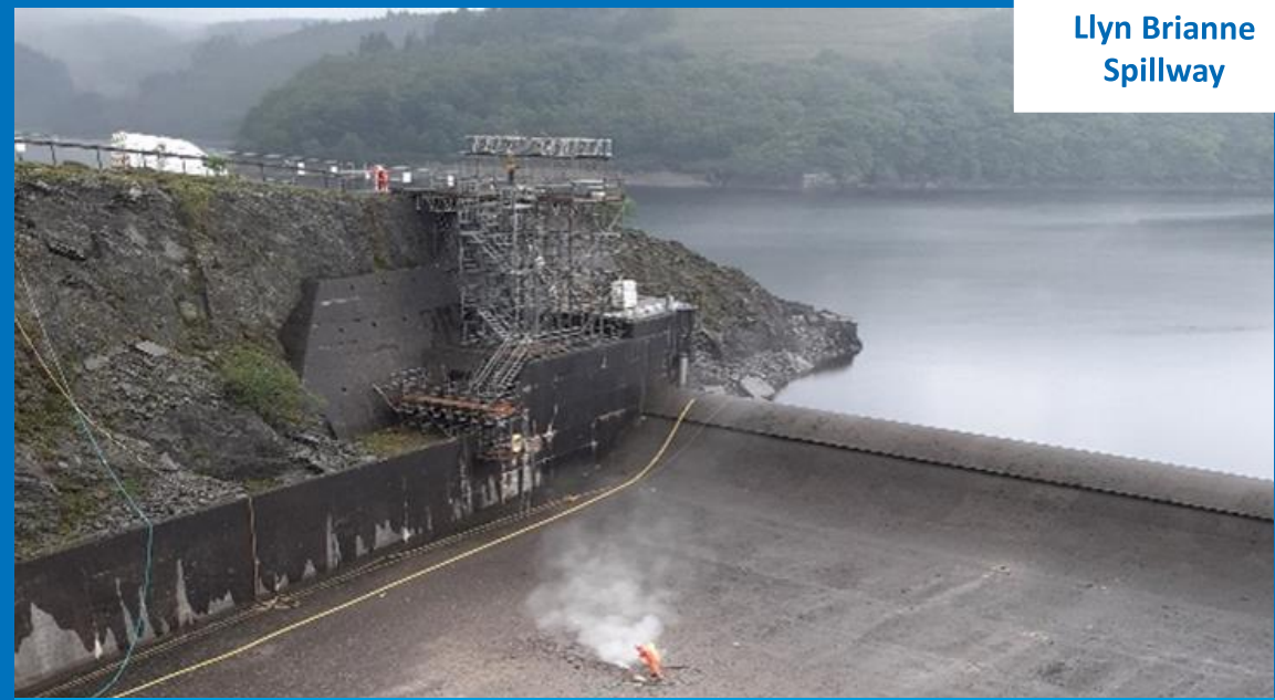
Concrete defect repairs on the invert and walls , (hydro demolition method used)
