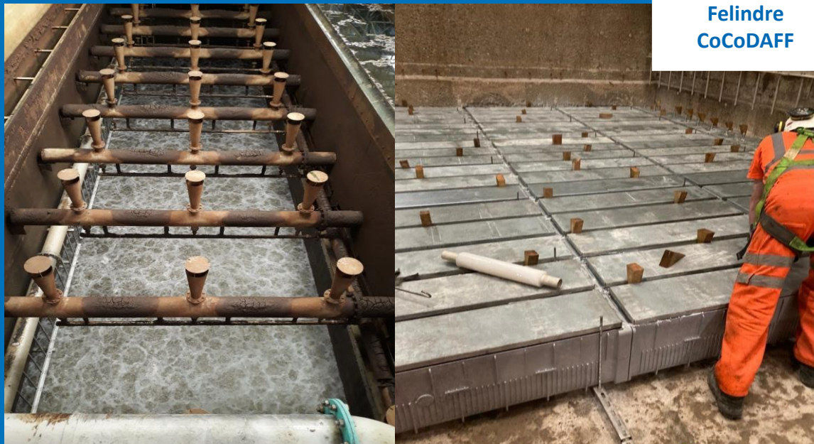
Filter E1 – Floor Replacement / Cap Installation and Pattern Test
