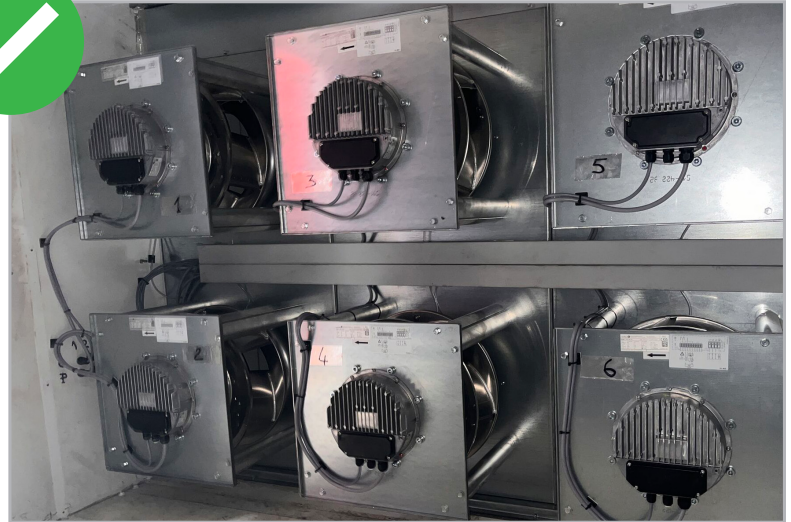
Efficient ECFanGrid as retrofit solution for the replacement of e.g. older belt driven fans. The ECFanGrid Retrofit KIT includes all mechanical parts: fans, cabinet, grid and screws.
