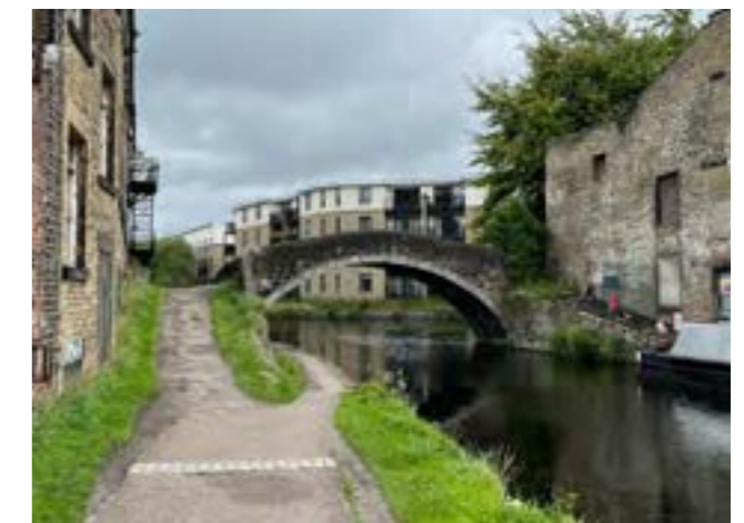
Listed Canal Bridge
