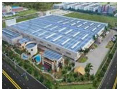
Figure 4 solar panels on the roof of the factory where PHOMI MCM is produced
