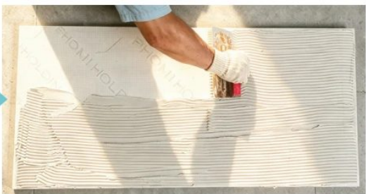
Apply specialized adhesive on the back of the product, ensuring full coverage rate > 90%
