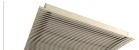
Aluminium roof frame
