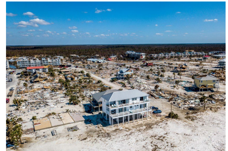
Florida home survives Hurricane Michael
