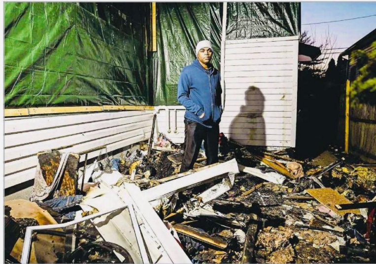
Omar Johnson stands in front of his former apartment in Elmont that was destroyed by a fire.
