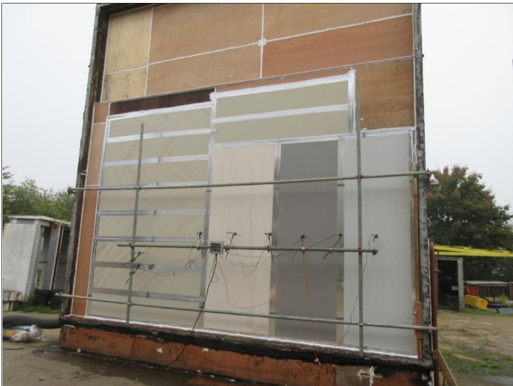
TEST SAMPLE DURING WIND LOADING
