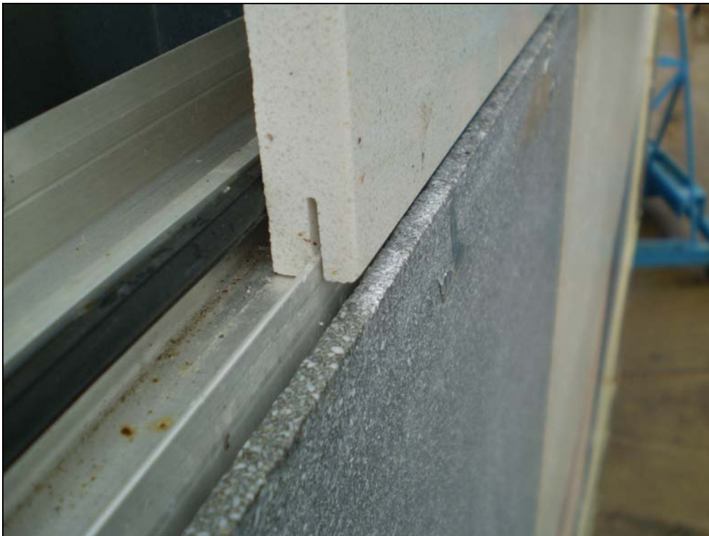
GROOVE IN EDGE OF TILE RESTING ON CARRIER FRAME
