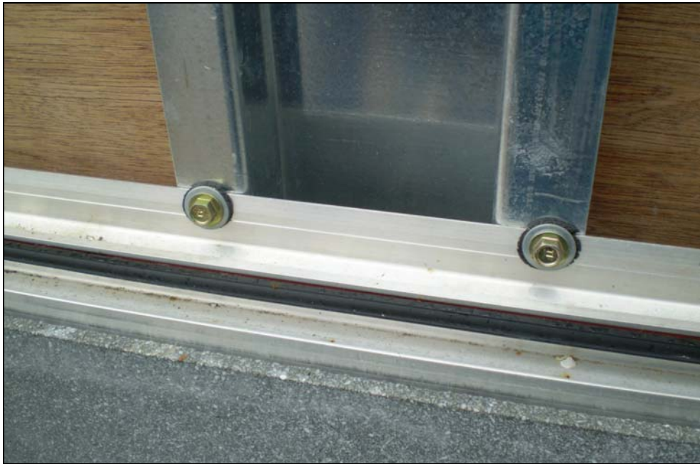
CARRIER FRAME FIXINGS INTO VERTICAL TOP-HAT SUPPORT
