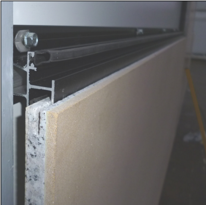
SUPPORT RAIL ALONG TOP OF PANEL
