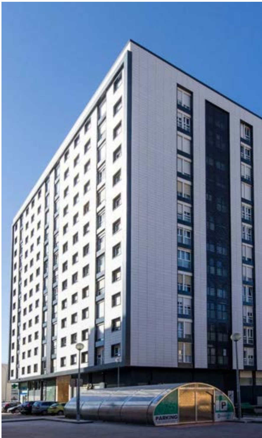
Refurbishment project, Torre Irrintzi, Pamplona.
