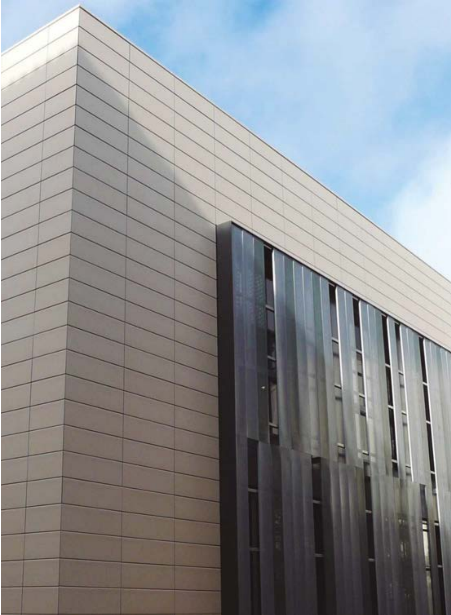
Solsona Residential building, Spain.
