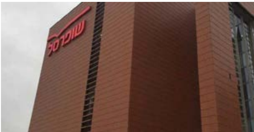
Logistics Centre Sufersal Project, Shoham High Park, Israel
