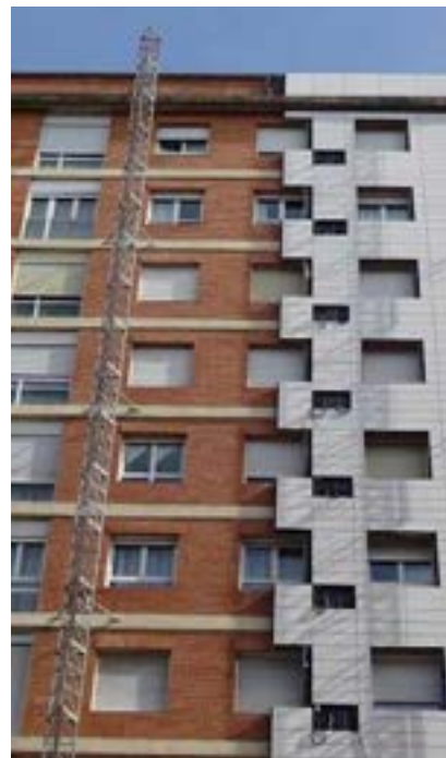
Photo of refurbishment.
