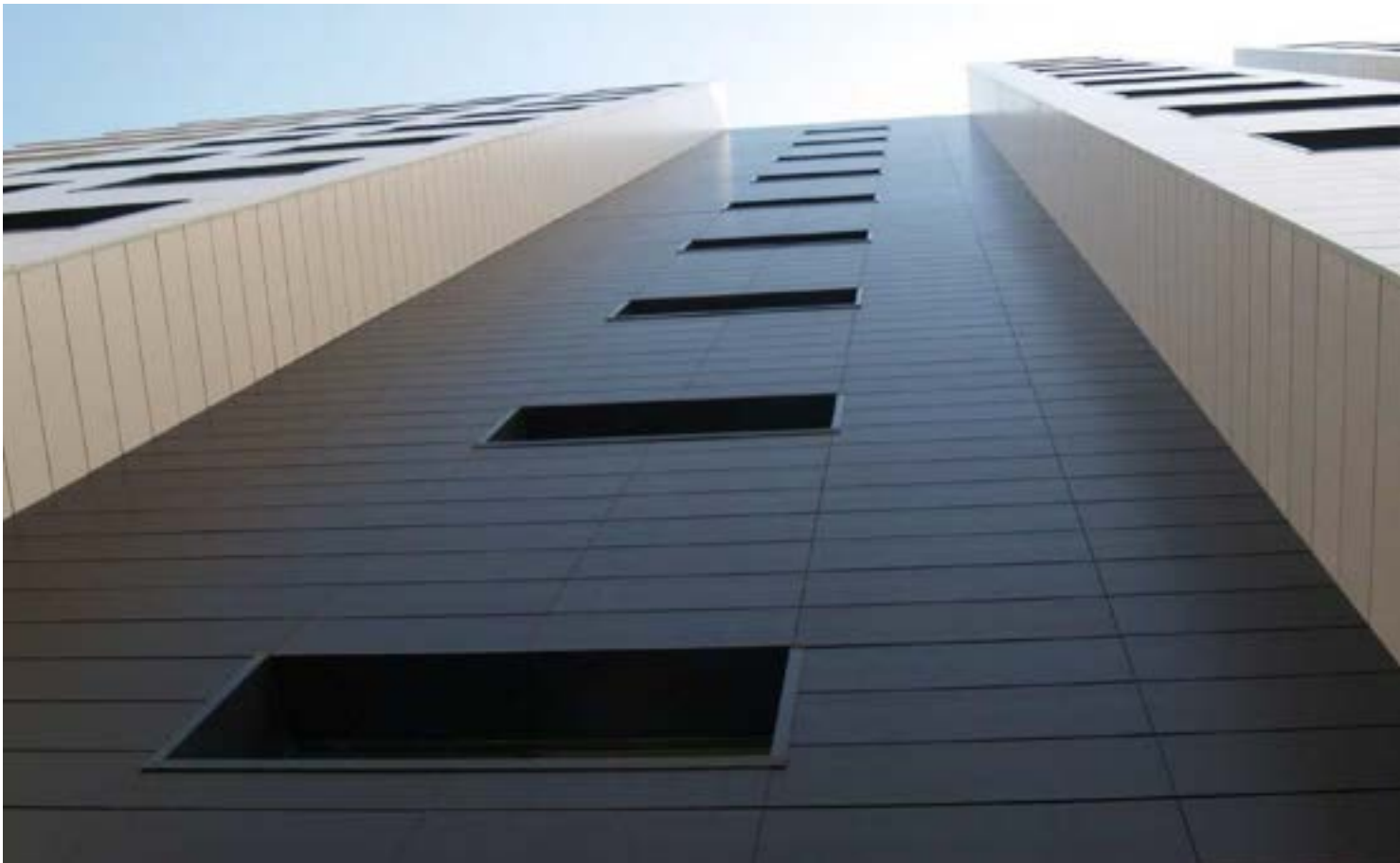
Burlada residential building, Navarra.
