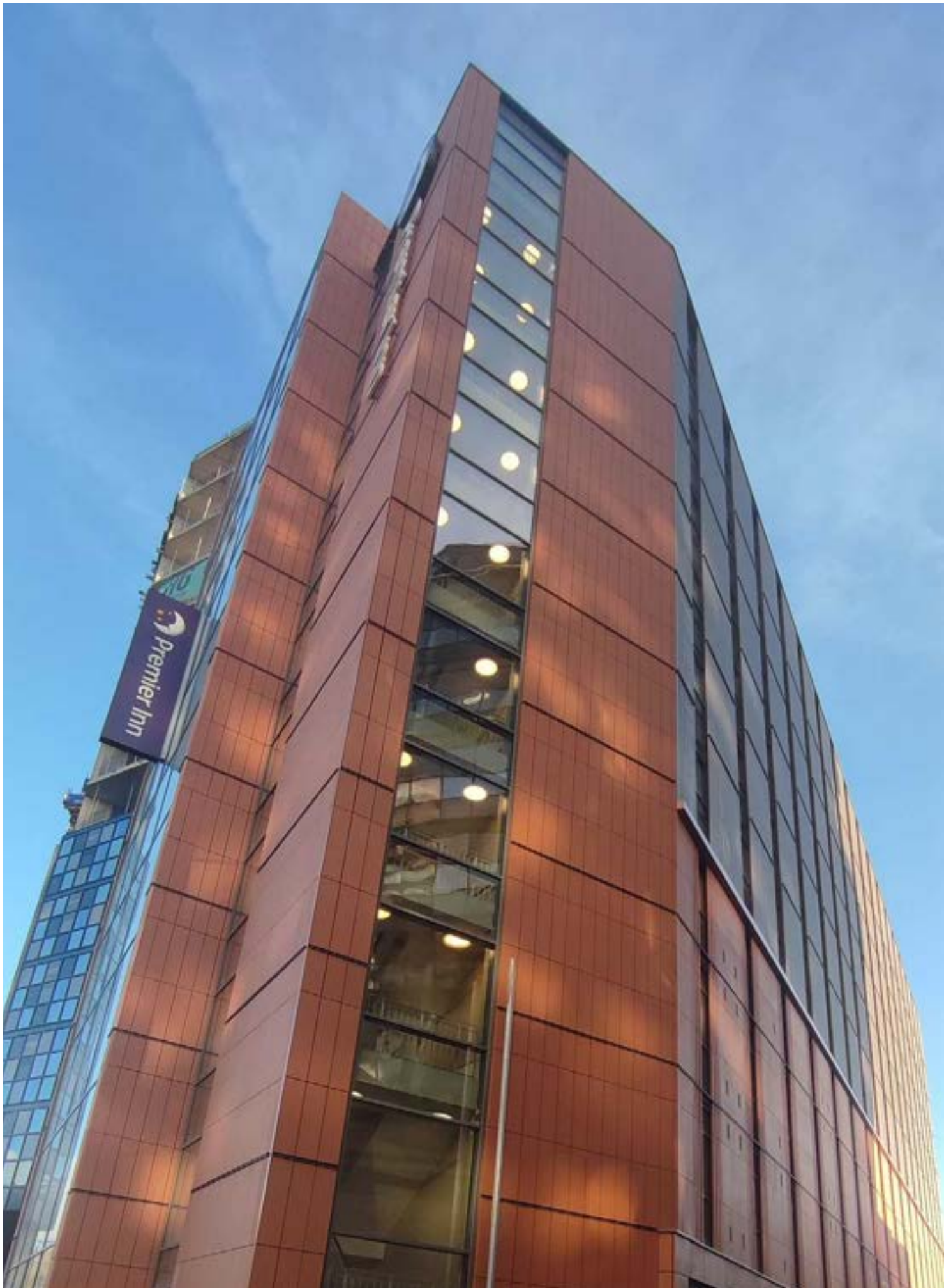
Hotel Premier Inn, Hammersmith, London, United Kingdom. Multifunctional UTM, square shutters and smooth panels of 1,200x600x40mm.
