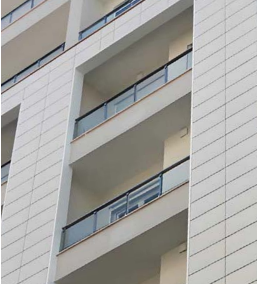
DITMAR FREDI BUILDING Tirana, Albania
