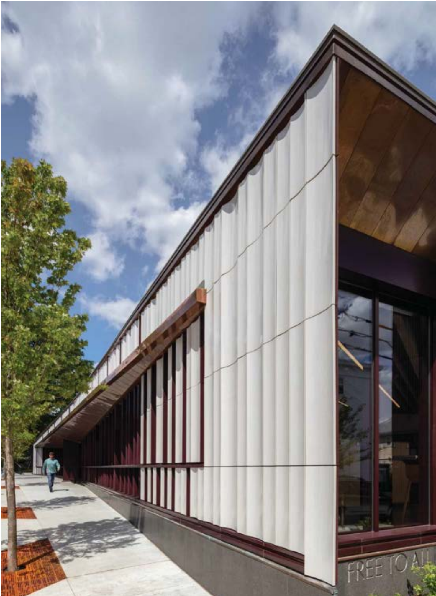
Boston Public Library, Adams Street branch, Boston, United States. Corner Curved detail PB and Curved PM.
