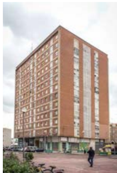
Torre Irrintzi before.
