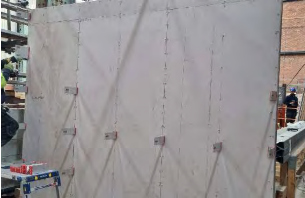
Plate 1 - Installation of Cement Particle Board and Helping Hand Brackets
