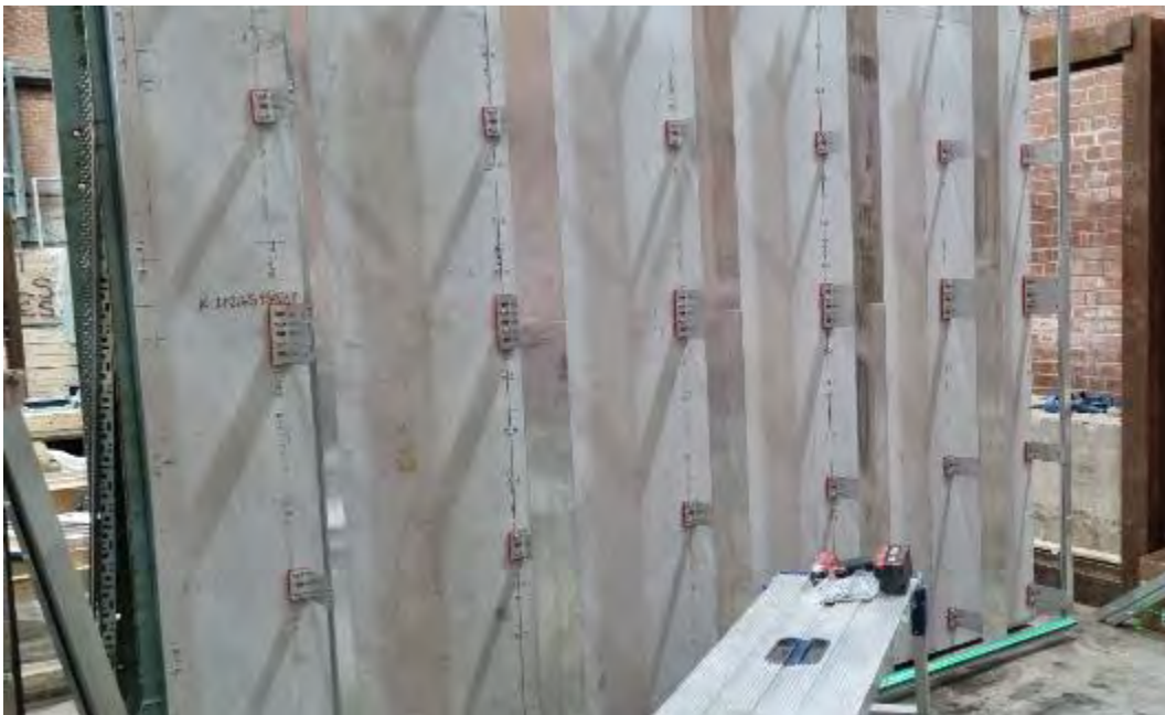
Plate 2 - Installation of 3 mm L-Shaped and T-Shaped Vertical Rails
