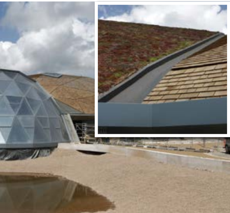
Club Kamikaze - Belgium RENOLIT ALKORPLAN Solar profiles as basis for a green wall
