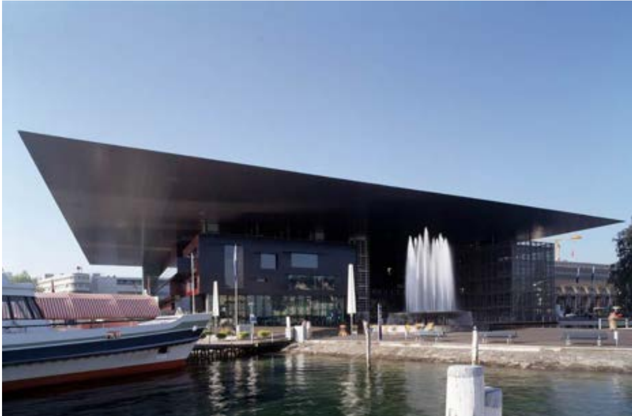
Roofing done with ALUCORE®
