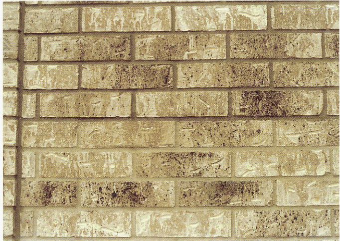
Fig. 5. The difference in mortar color in this example was determined to be the result of a change in both sand and type of cement used in the mortar.
