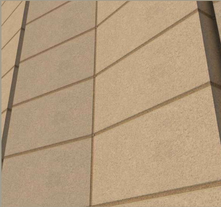
ABRI Pattern: Opposed Wedges Stack Bond – horizontal
