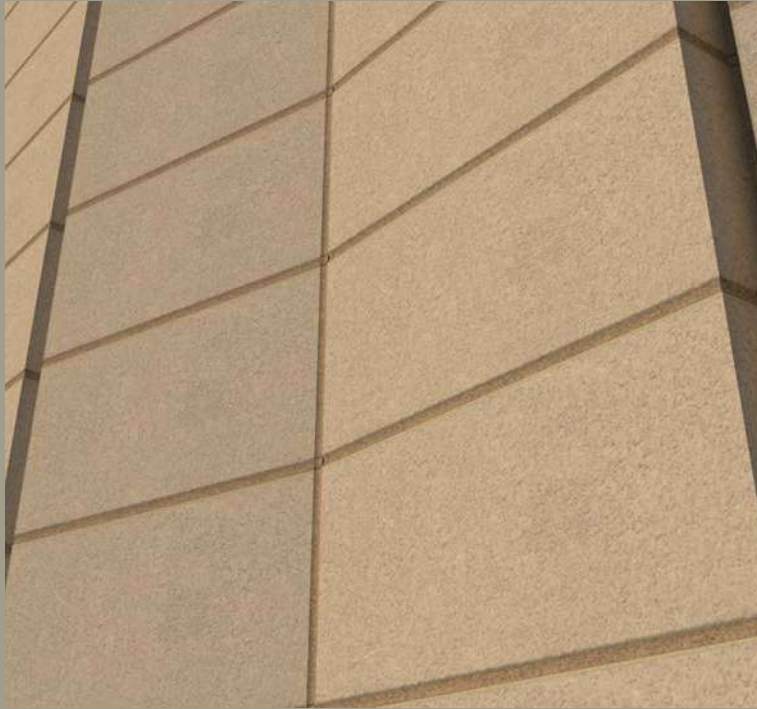
ABRI Pattern: Opposed Wedges Stack Bond – horizontal
