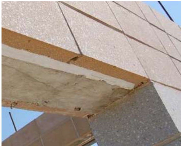
HI-R reinforced as lintel after grout has cured and wood forms have been removed
