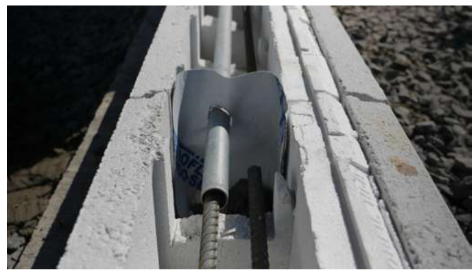
Bond break at control joint
