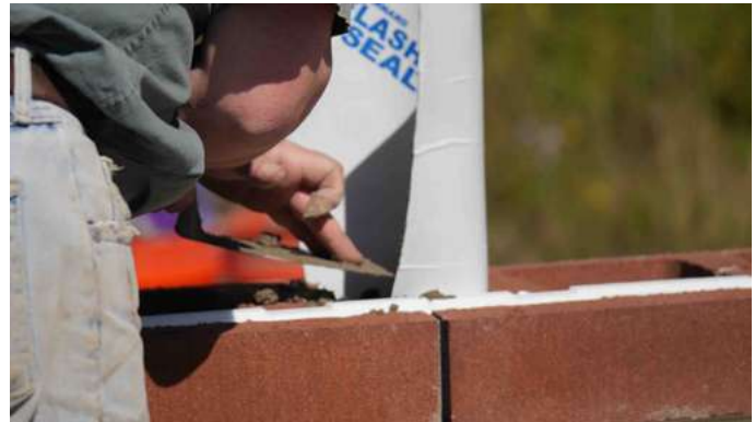
Bond break at control joint
