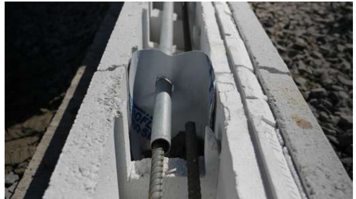
Bond break at Control Joint
