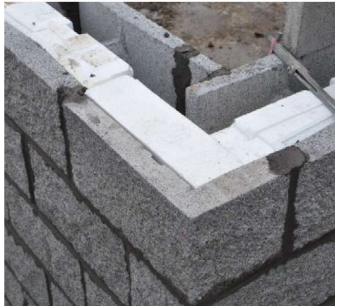
Corner with L-shaped fitting cut from CMU and soap. The face shell of the HI-R-H unit to the right can be cut as needed to accommodate horizontal reinforcement
