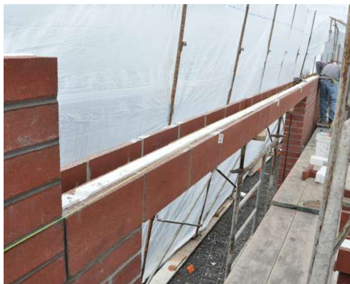
HI-R/HI-R-H Closed Bottom Lintel – Pre-fabricated installation
