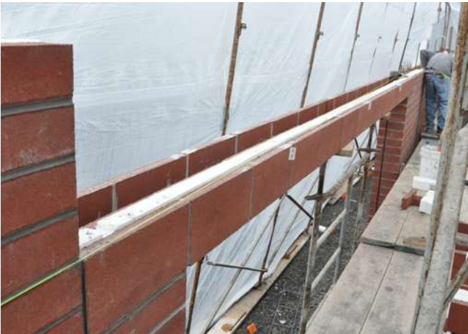
HI-R/HI-R-H Closed Bottom Lintel Pre-fabricated installation
