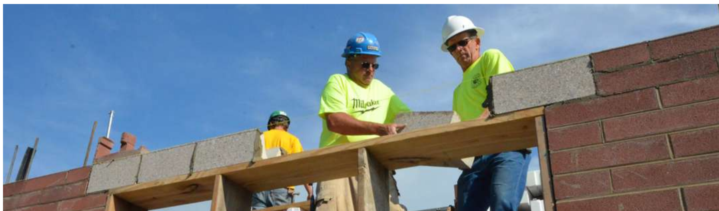
Traditional masonry lintel installation using a form (this lintel is not insulated)
