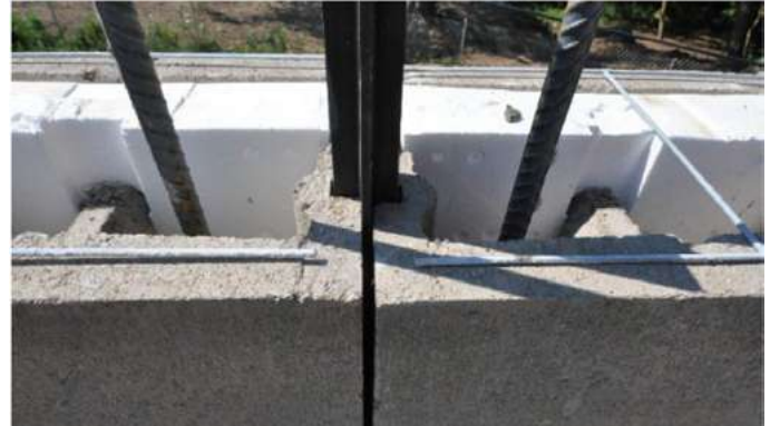
Control joint using HI-R-H Sash/Jamb Unit
