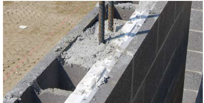
Partially Grouted HI-R Wall
