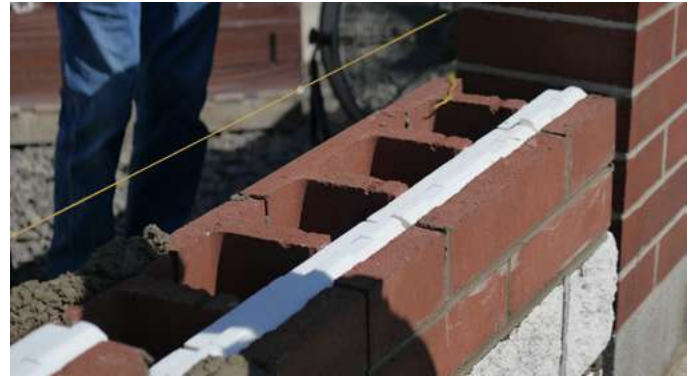
HI-R Half High Wall Under Construction
