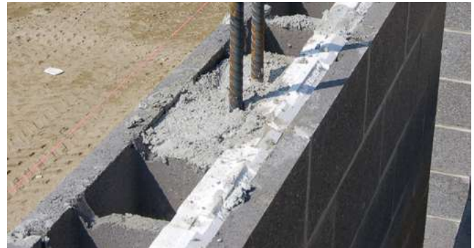
Partially Grouted HI-R Wall (shown with 12×8×16 unit)
