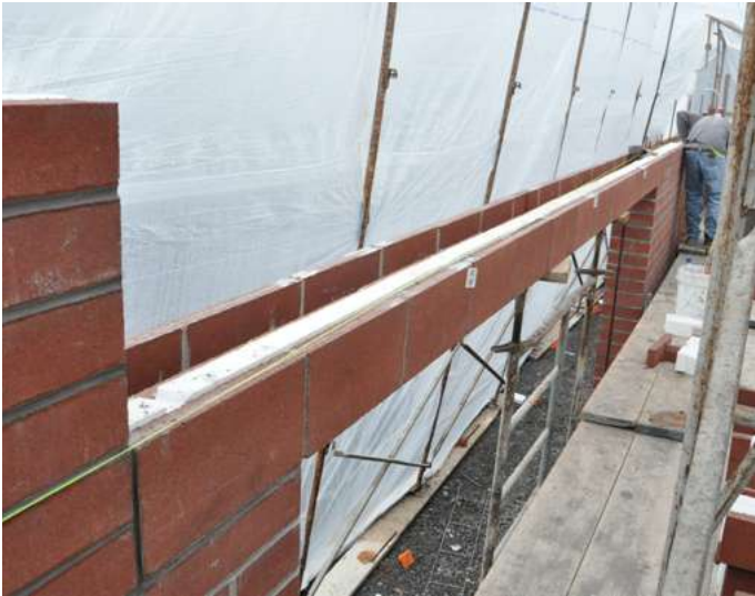
HI-R/HI-R-H Closed Bottom Lintel – Pre-fabricated installation
