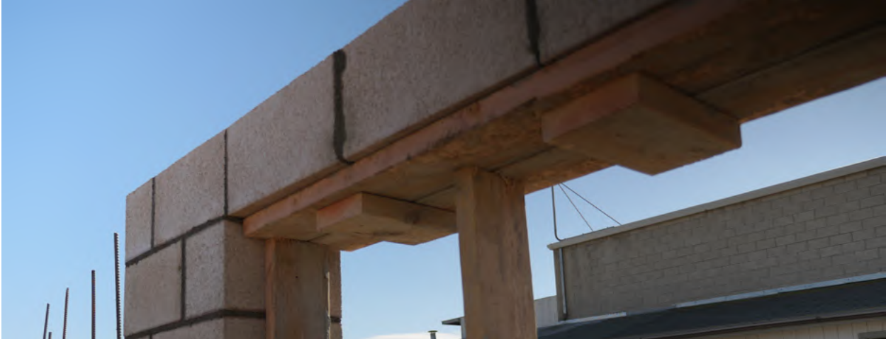
Lintel using HI-R-H Units shown under construction
