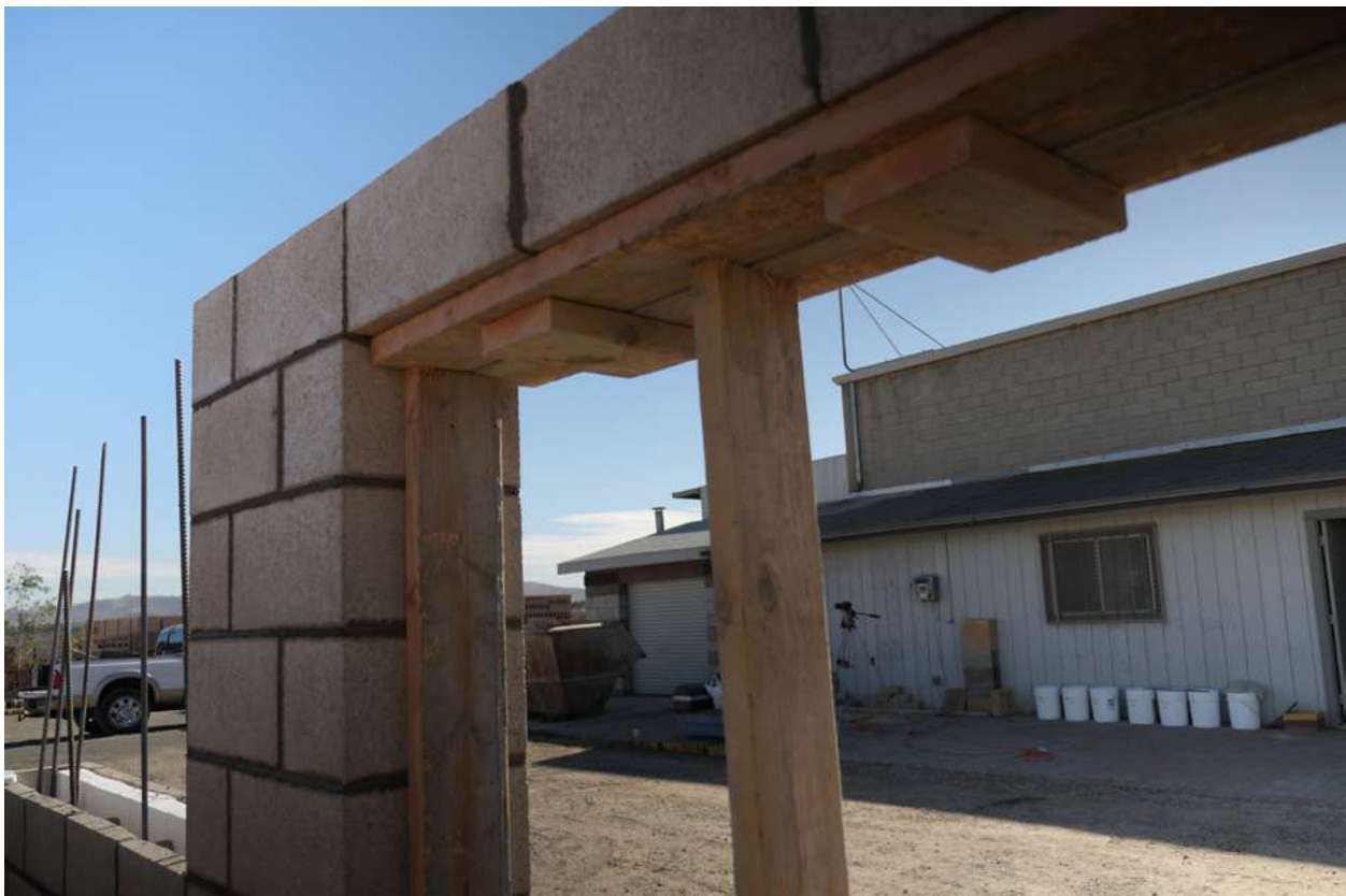
Forms supporting lintel during construction (shown with HI-R-H units)
