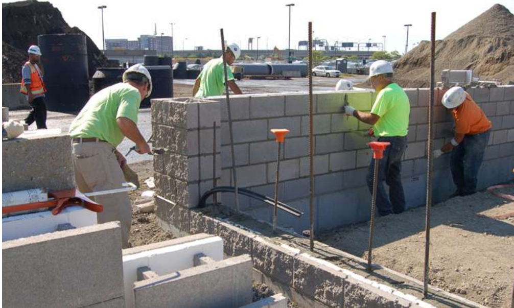
HI-R Bond Beam, Corner and Control Joint Under Construction
