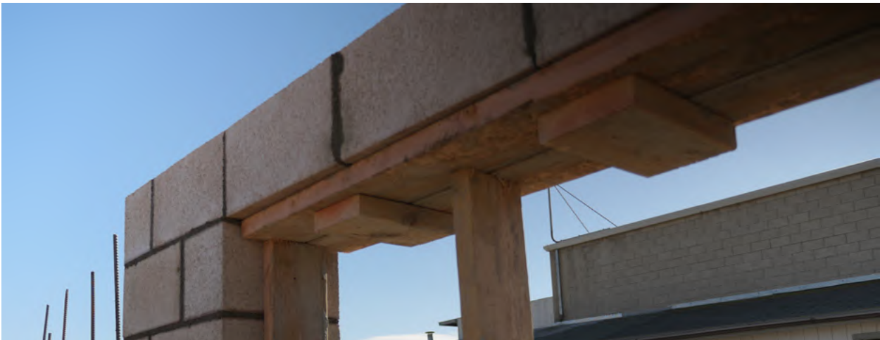
Building a lintel on a form – pre-fabrication is also an option
