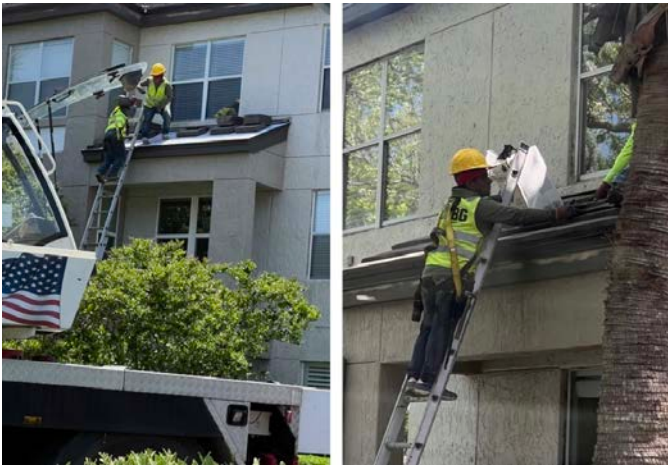
Work on other rooflets
