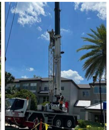
Loading roofing tiles and the crane that would lift the container to the roof
