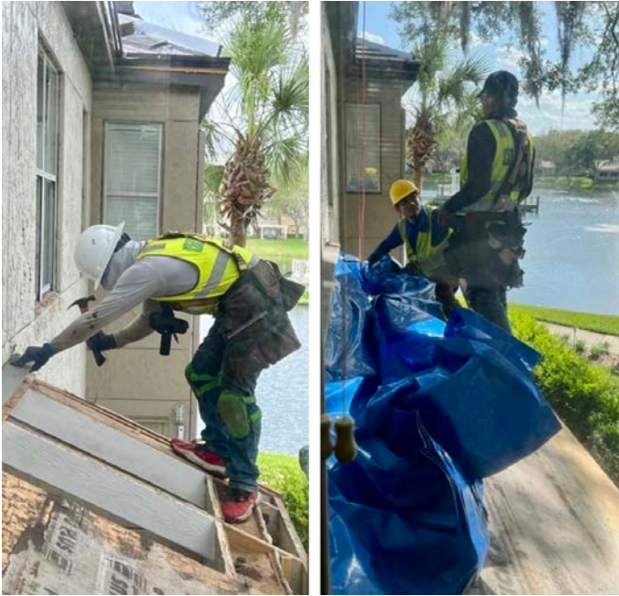
View from Payne's apartment of work on a rooflet
