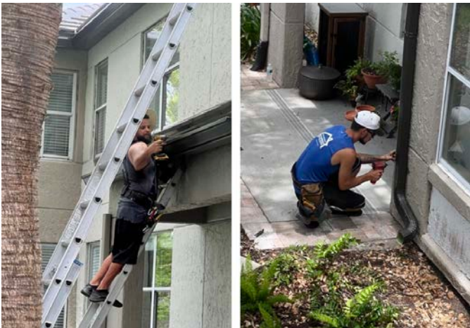
Gutter and drainpipe replacement
