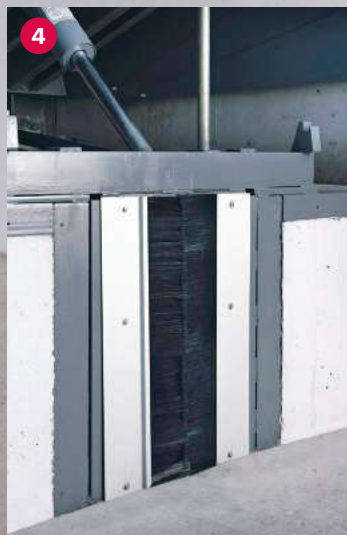
Clean dock face
