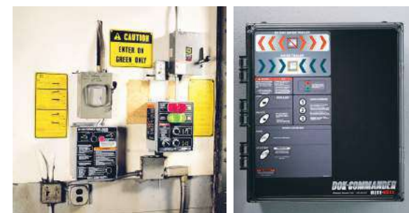
Multiple controls at each dock position can be complicated and potentially dangerous.
