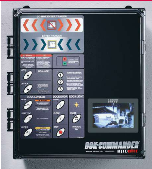
Rite-Hite Dok-Commander offers simple access to controls for each dock component.
