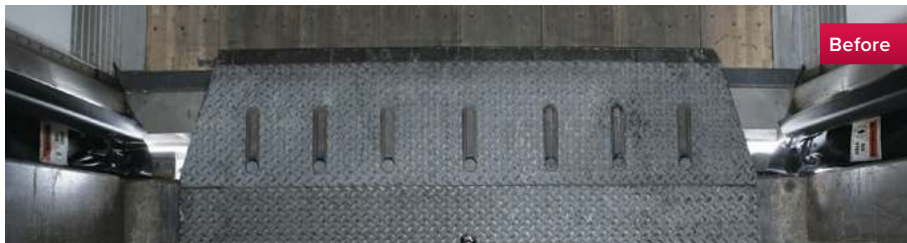
Open gaps at dock leveler corners allow unwanted elements to enter and expensive energy to escape
