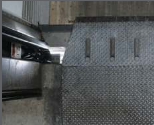
Beneath and around dock leveler
