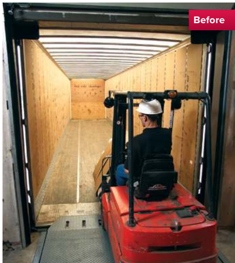
Exposed trailer door hinge gaps
