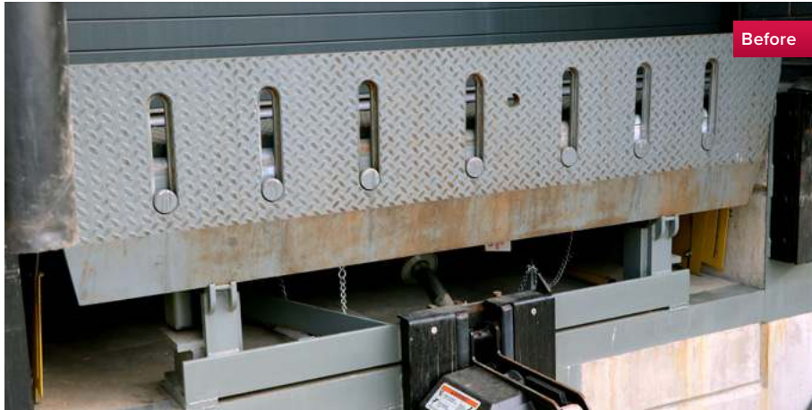
Open dock leveler pits invite the infiltration of bugs, dust, pests and debris
