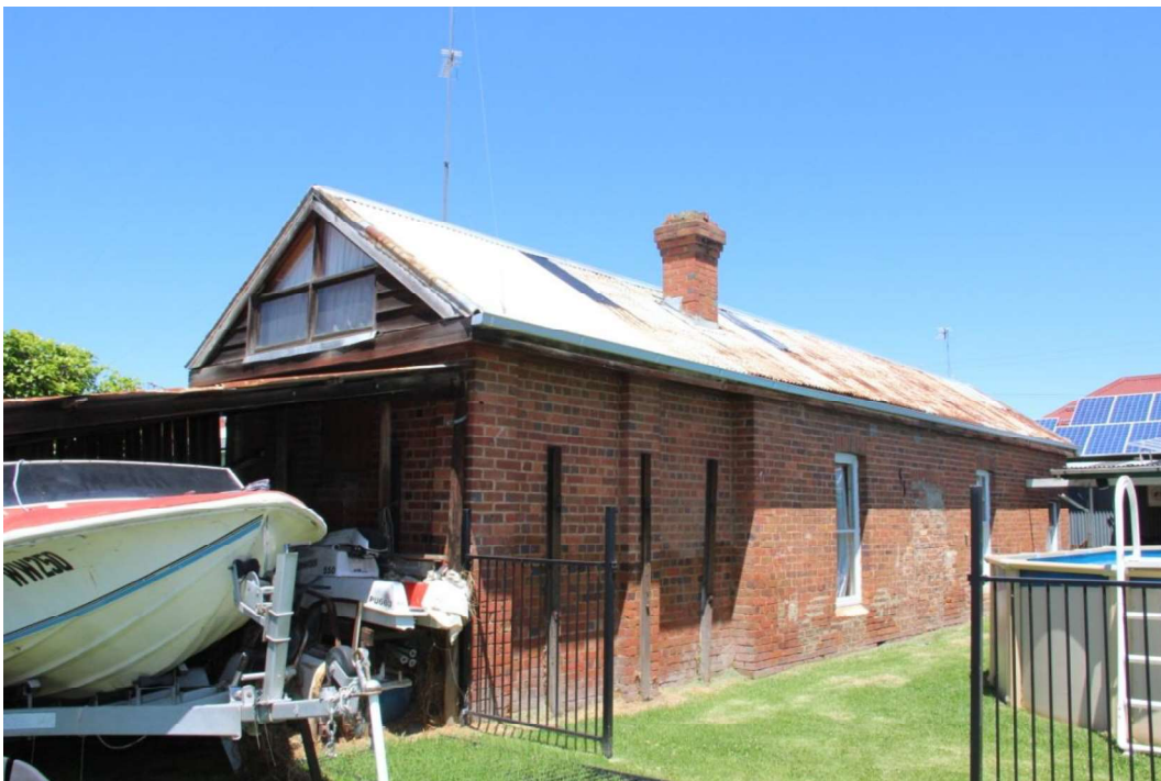
Figure D7. The north and east elevation of the 1902 brick bakery. A corbelled brick chimney remains on the northern roof plane. The north and east elevations of the bakery remain face-brick. The north end of the east elevation has recessed planes reinforced with early timber supports (that supported the weight of the sand on top of the oven). The north elevation originally had four openings, all with radiating brick voussoirs above.
