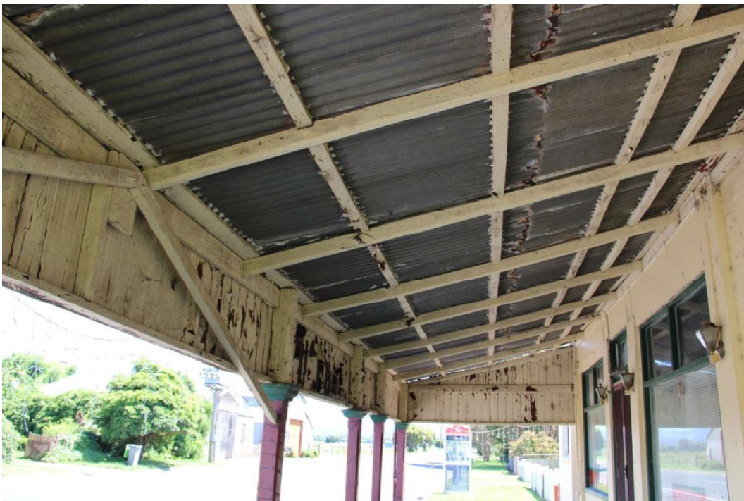
Figure D3. The verandah to the store has a skillion-roof clad with corrugated iron, supported by large stop-chamfered timber posts with timber capitals (on a tall modern concrete base). The original timber frame is evident underneath. The top section of vertical timbers (sign board) to the sides of the verandah are original, the rest is a later addition.
