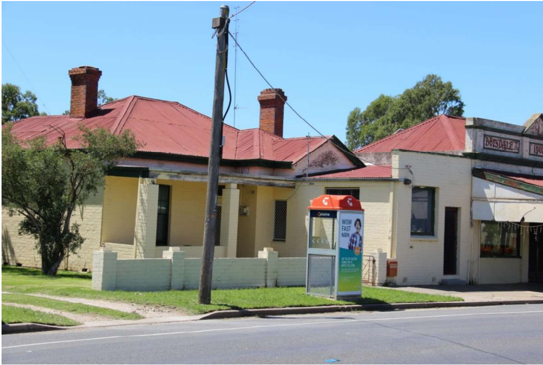
Figure D4. The residence has a hip-and-gable roof clad in corrugated iron and retains two corbelled brick (unpainted) chimneys. A small brick addition with a skillion roof projects off the store, with a simple brick parapet to the south end of the facade, essentially extending the facade of the general store (dates to a later period).
