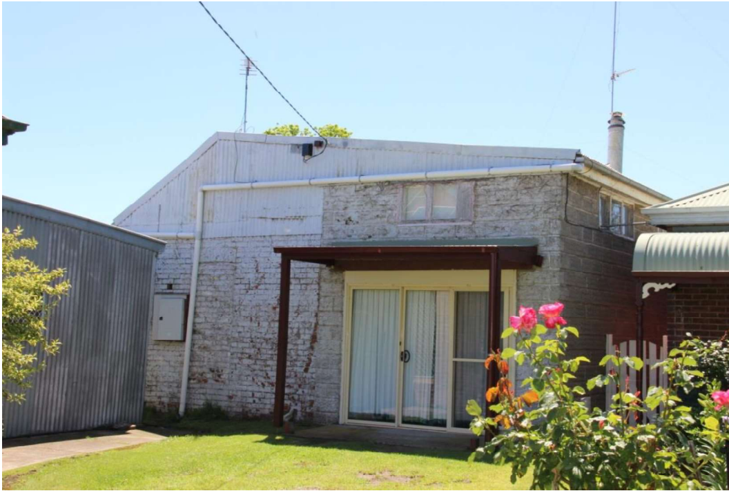
Figure D6. The front elevation of the bakery, as seen from the street, unfortunately shows the large addition and painted 1902 elevation. The addition to the south is constructed of vermiculated concrete blocks.
