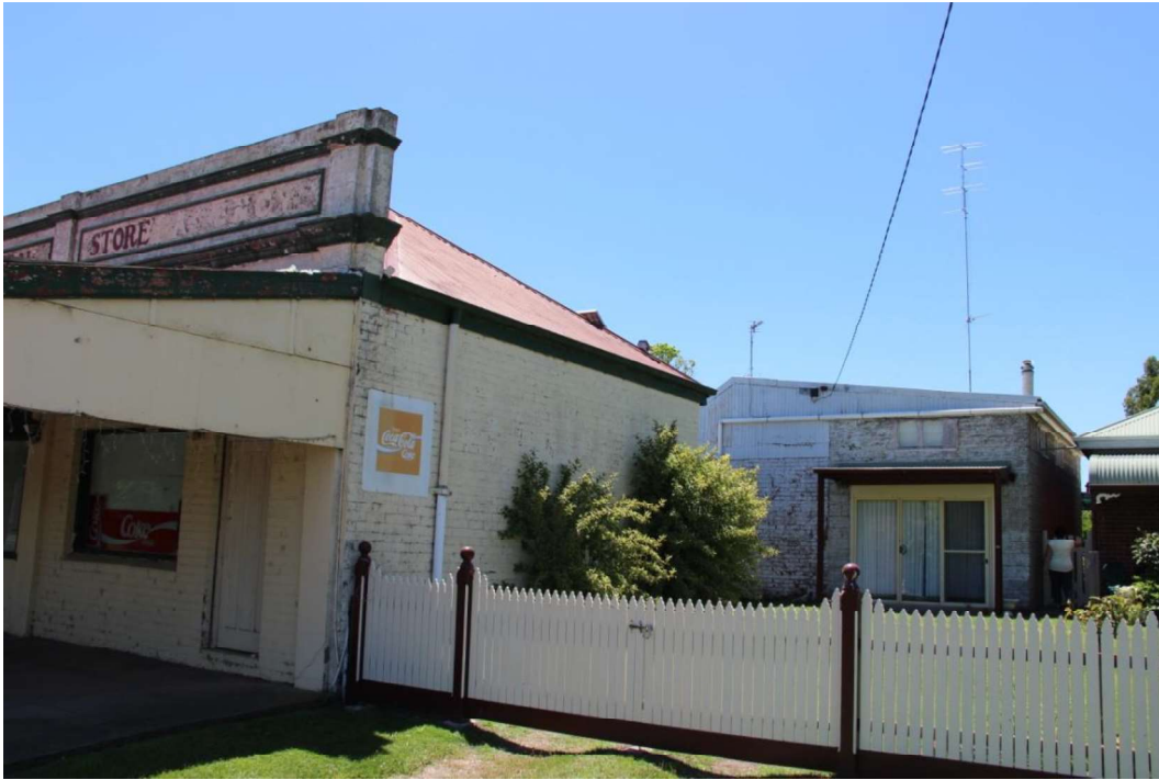
Figure D2. The general store on the front title boundary and the bakery (overpainted with a modern addition) painted white to the rear (east).
