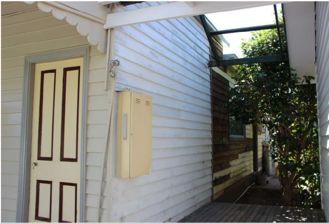
Figure D3. The south elevation has no windows to the original c1891 section. To the rear is a modern weatherboard addition.
