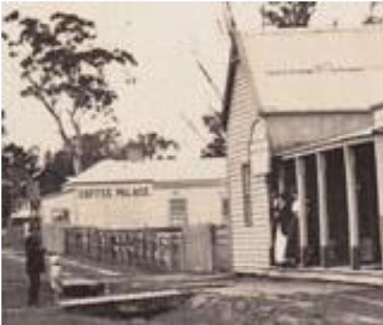
Figure H1. An early photo (date not known) shows the weatherboard building in the background, at a distance from the south, with ‘COFFEE PALACE’ painted on the south elevation of the front section. The section to the rear had two openings (MDHS, ID. P03799VMFF).
