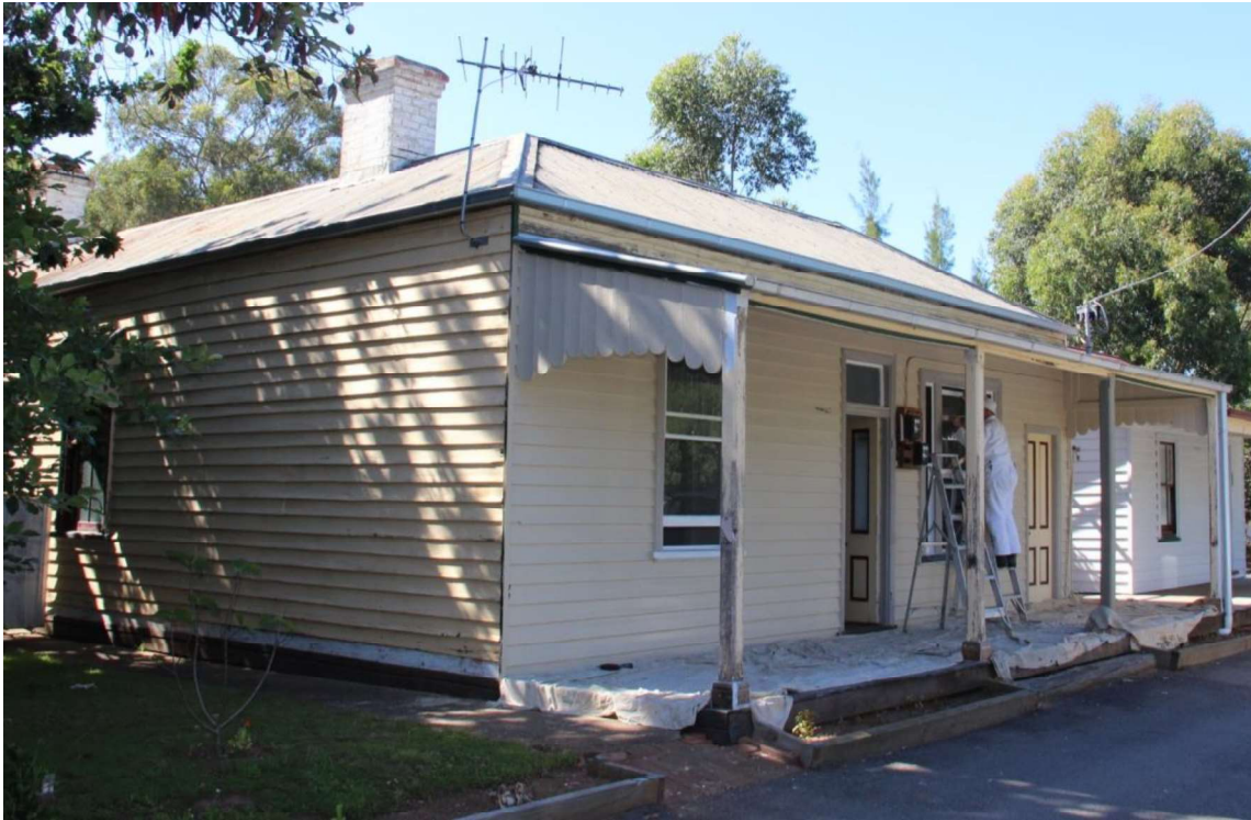
Figure D1. The asymmetrical facade has a skillion-profile verandah clad with (recent) corrugated iron and timber (round-edged) palings to the sides, supported by stop-chamfered timber posts with timber bases. The facade has a central entrance, two different types of windows and a second entrance at the southern end.
