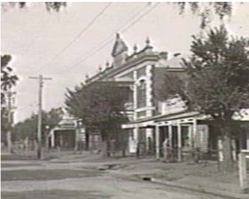
Figure H2. A photo dating to 1932 that showed the hotel from a distance, from the north-west. The quoining to the corners was painted bright white and atop the parapet was the pediment,
