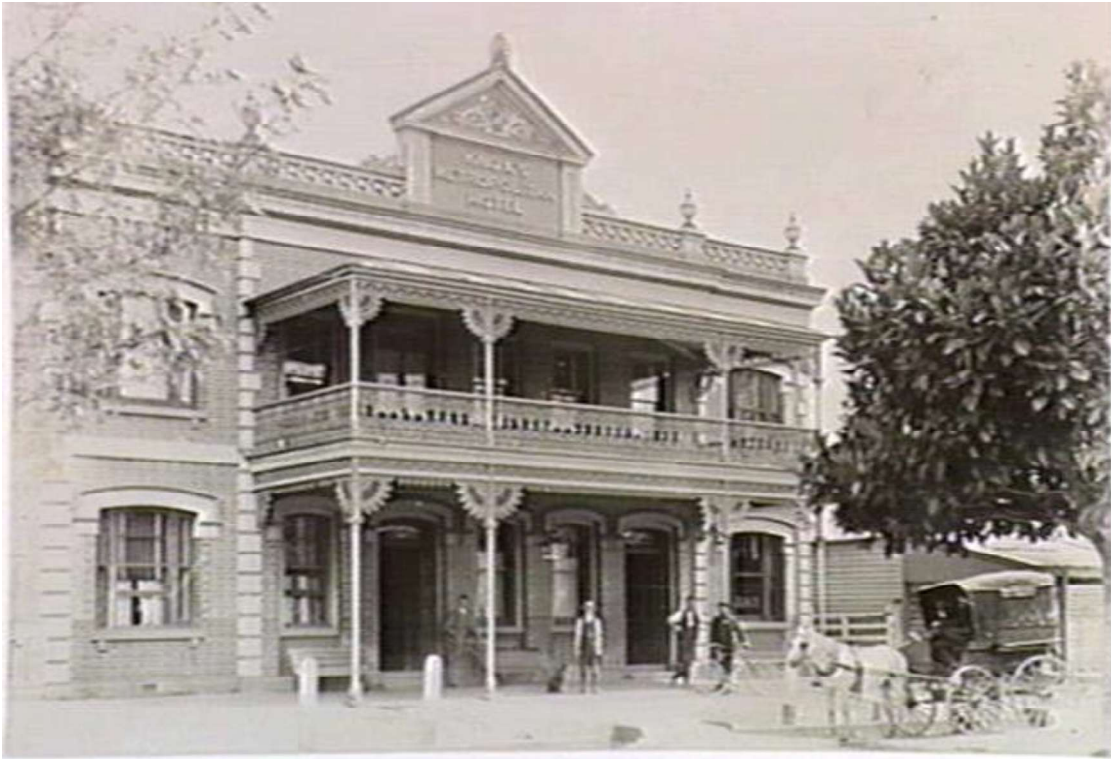
Figure H1. A photo dating to 1910 that showed the facade of the hotel. The parapet had urns atop each pier, while the pediment read '[indecipherable owner's name] Metropolitan Hotel'. The two-storey verandah had an ornate balustrade, a frieze to both floors, and round brackets to each supporting post (SLV).
