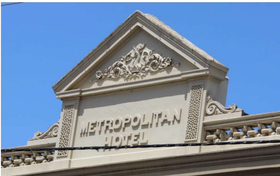
Figure D1. The two-storey building was constructed of brick (overpainted), with tuck pointing to the facade, on a rendered plinth. A decorative parapet to the facade stops at a pediment. The pediment sits central over the two-storey verandah below (reconstructed in 1996).
