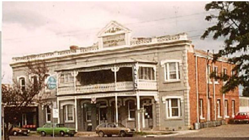
Figure H4. Barrett's Metropolitan Hotel (c1970s-80s) showed the facade and west elevation when it remained face-brick (NT).
