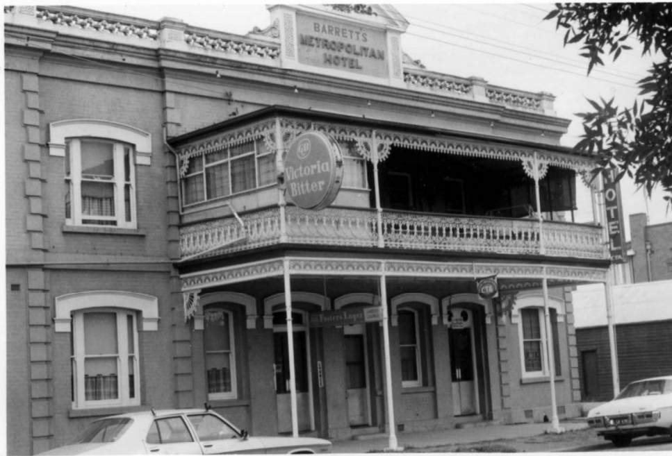
Figure H3. A photo dating to 1970 that showed that the pediment now read 'Barrett's (painted) Metropolitan Hotel' and that the urns had been removed by this date. Some of the round cast-iron brackets to the ground floor had been removed by this date and the verandah to the first floor had been in-filled at the east end (SLV).
