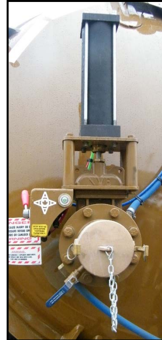
Green indicator (appears when valve in “open” position)
