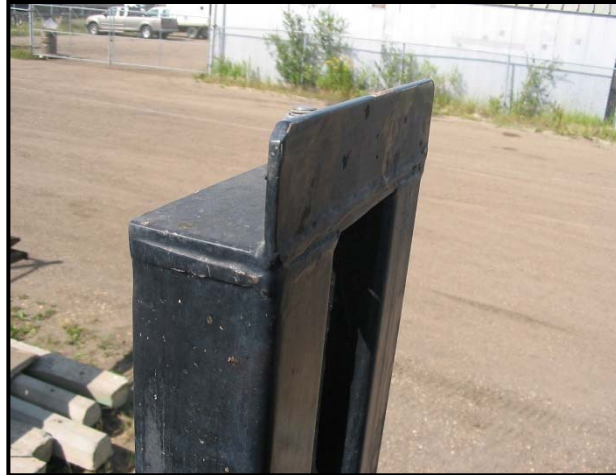
Plate Atop Main Frame Column that Receives Locking Bracket
