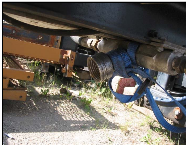
“T” Connection Below Spool
