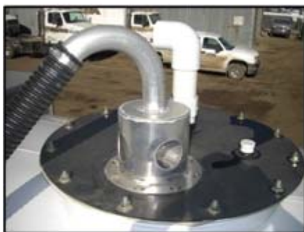
Tank – Top View
