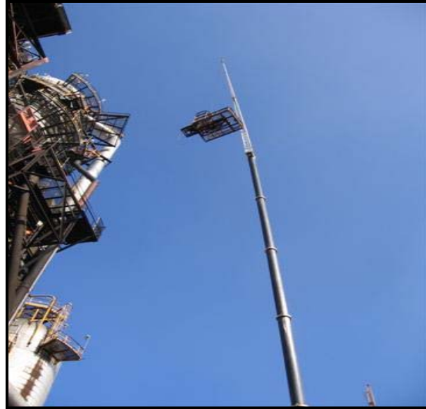
Crane Lifting Snout Lance
