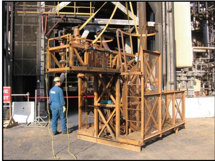
Snout Lance Unit Preparing for Rigging
