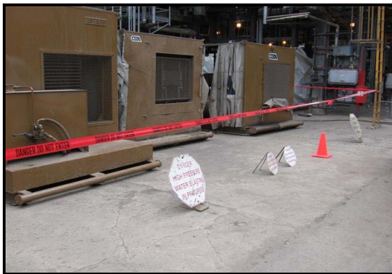
Front View (area flagged and tagged)
