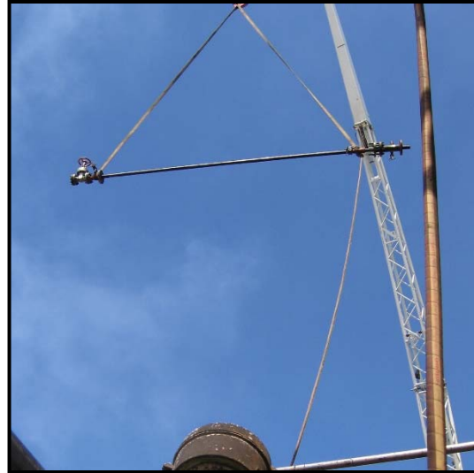
Crane Lowering Shroud To Platform
