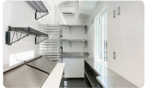
Kleenclad™ hygienic cladding — installed
