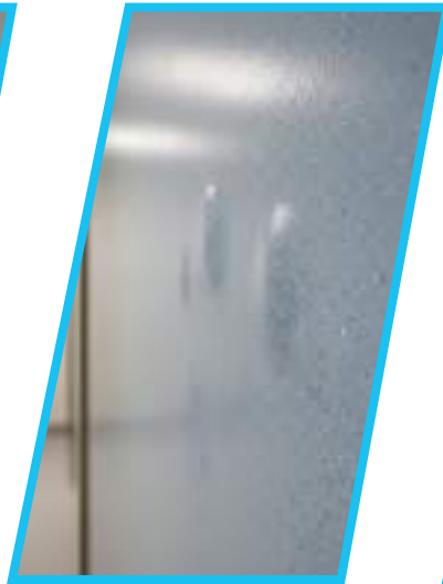
Wall Vinyls – Surface Undulations, Bubbling and Peel Off
