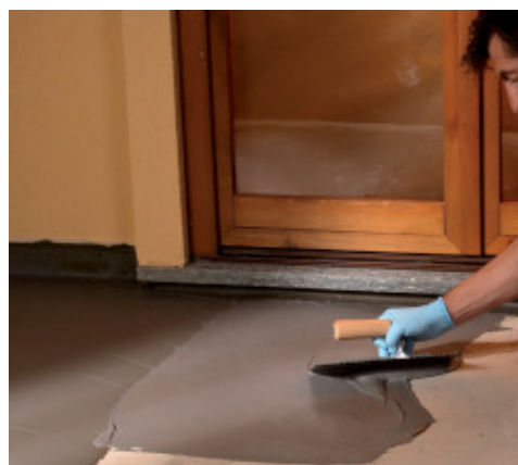
Waterproofing of terraces by trowel
