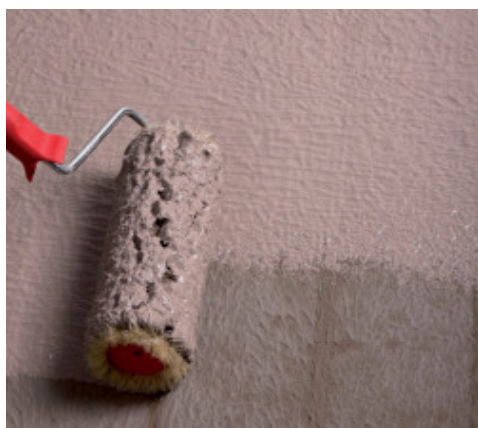
Waterproofing of terraces by roller
