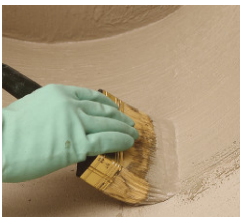
Waterproofing of details by brush
