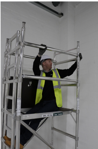
7. Sitting through the trapdoor fit 4 horizontal braces to the verticals above each rung of the frames above the platform to complete a guardrail.
