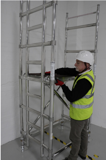
5. Add temporary trapdoor platform to the 3rd rung, trapdoor at the ladder end.
