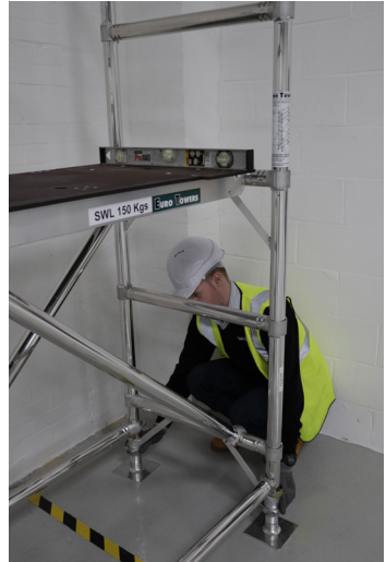
6. Level the tower adjusting the leg nut using a spirit level as a guide.
