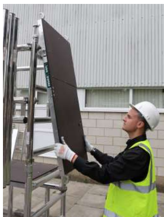
16. The platform can be located on the opposing side of the tower from the frames.
