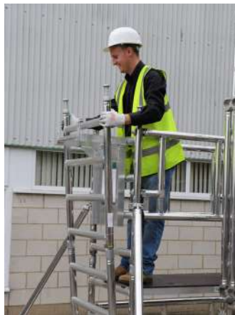
21. Retrieve a set of frames from the side assembly bracket and fit.
