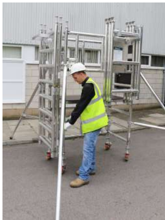
19. Re-Fit 4 stabilizers, one on each upright of the tower if this was not already done.
