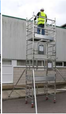
3.1m Tower Set up
