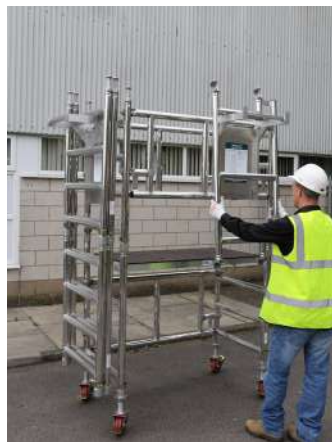
15. Stow 3 guardrail frames on the front assembly bracket.
