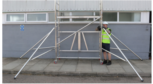
6. Fit 4 stabilisers at earliest opportunity keeping lower arms as horizontal as possible ideally 45 degrees. Stabilisers are fixed onto the frame uprights in each corner by the attached couplers.
