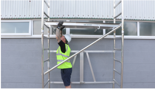
5. Fit your trapdoor platform to the 7th rung.
