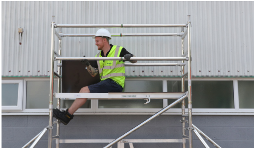
7. Fit 4 horizontal braces to form a guardrail in the seated position using the 3T Method (Through The Trap). Position above the 10th rung and below the 9th using the locator nut. For builds 1.8m and below, go to step 12.
