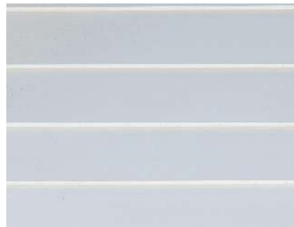
Cladding - James Hardie Weatherboard
