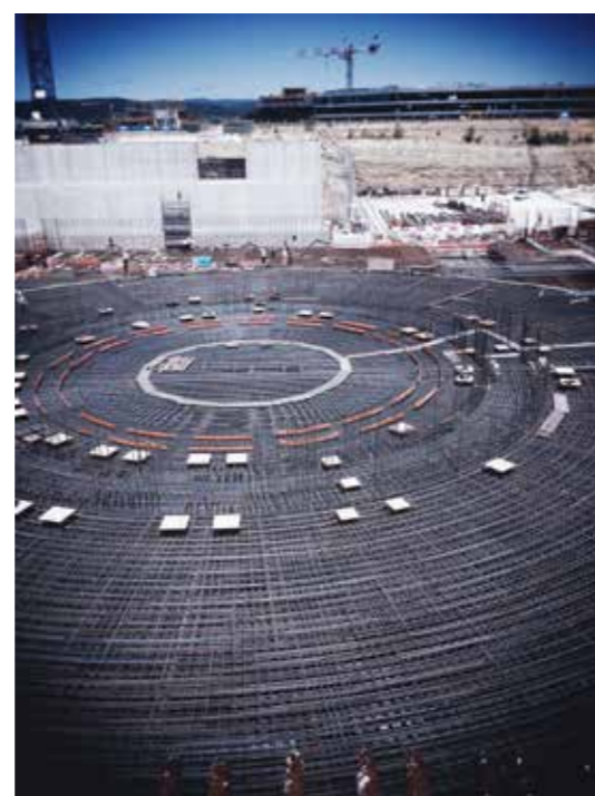
The tokamak pit of ITER some years ago. Pictures: Eyesteelfilm
