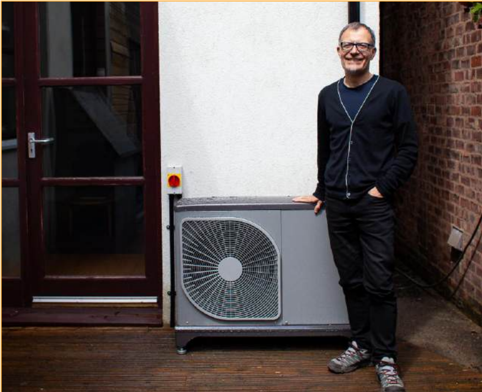
It's possible to fit heat pumps on terraced homes where neighbours are close - though it's easier if a smaller heat pump is needed such as the 6kW unit shown here.
