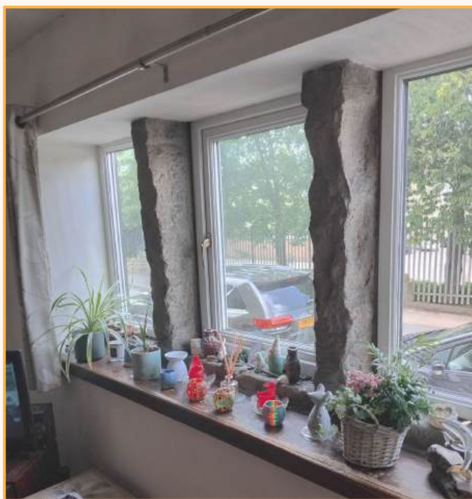
Photo: stone mullions to windows.
