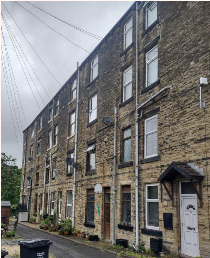
Entrances and ground and first floors to 'under dwellings' with two storeys of 'overdwellings' accessed from the opposite side above. Photo credit: A Gardner
