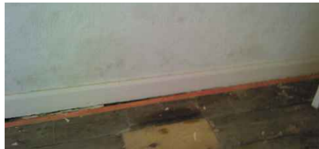
Exposed floor slabs showed colder temperatures and more air leakage than those with floor coverings.
