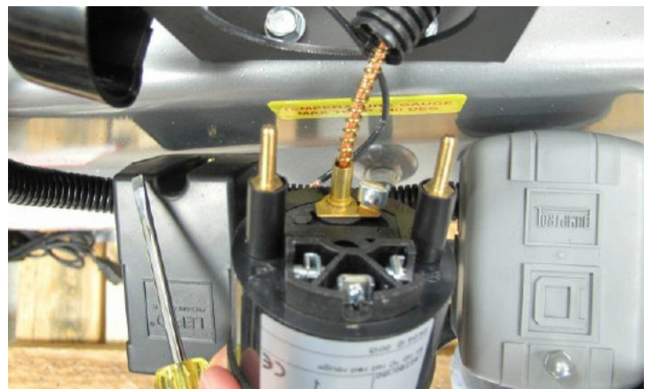
Wires removed from old switch
